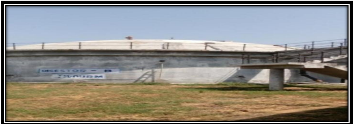
Fig 5.2.10 Sludge digester tank
