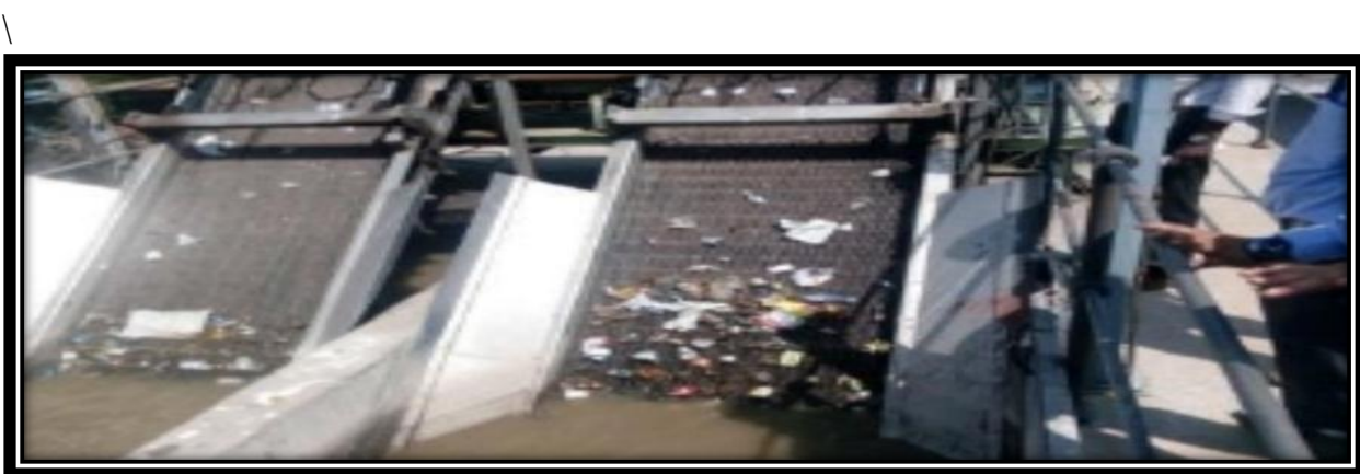
Fig 5.2.6 Showing automated screening
